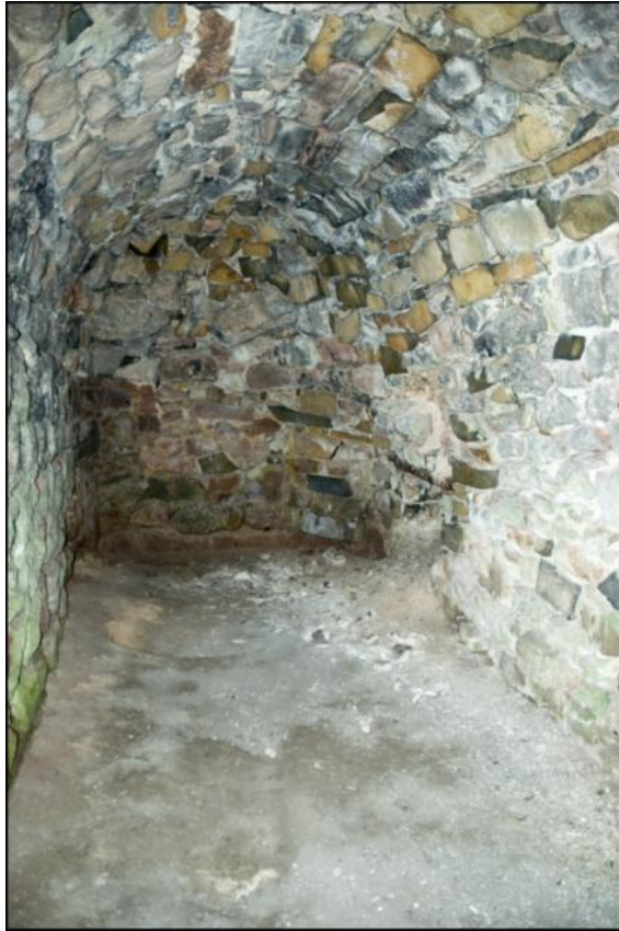
Plate 7, the interior of one of the west kiln discharge chambers
