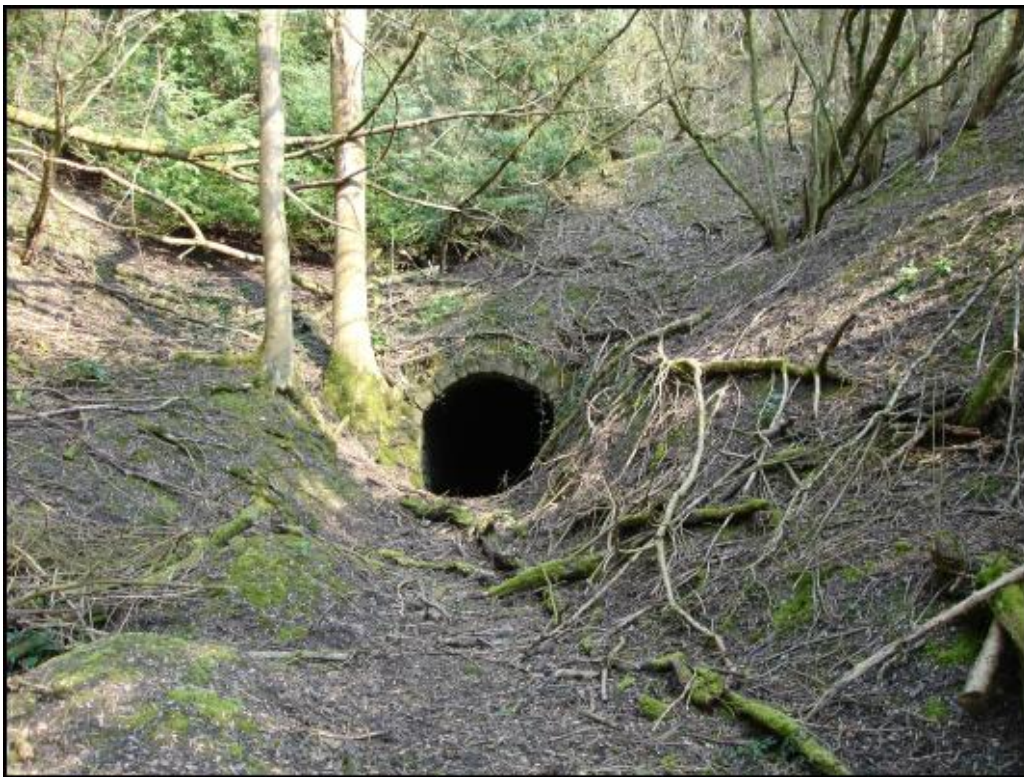
Plate 3, The drift mine entrance
