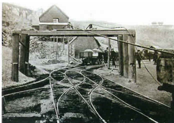
Right: Top of the incline from where loaded trucks were released. In the background is the drum house from which ran the wire rope to be attached to the trucks.
